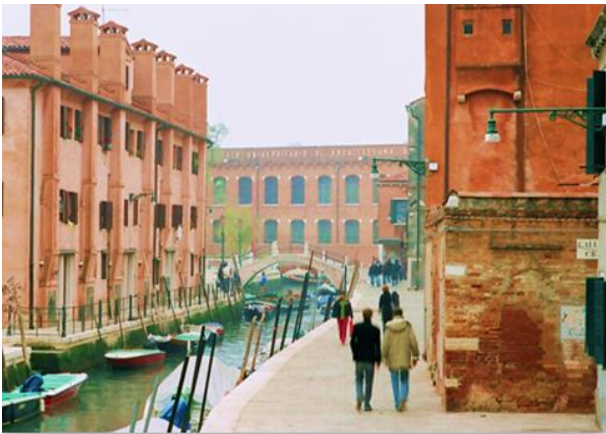
The “Cotonificio Veneziano” building of IUAV
